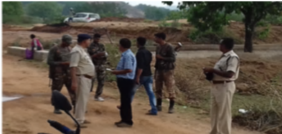
Figure 12. Armed police protection to engineer constructing the haul (coal transport) road at Jugra village
