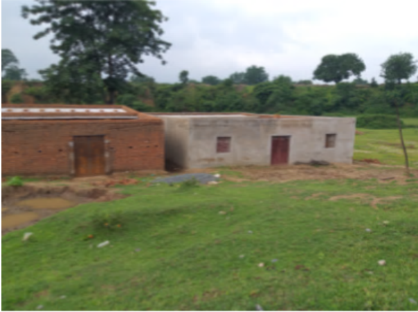
Figure.7. New houses built by evictees at Itiz village in proximity of Pakri-Barwadih coal mines.
